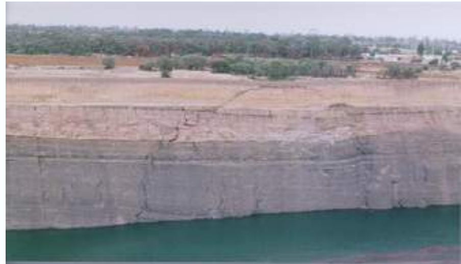
Panel failure – Mine B
