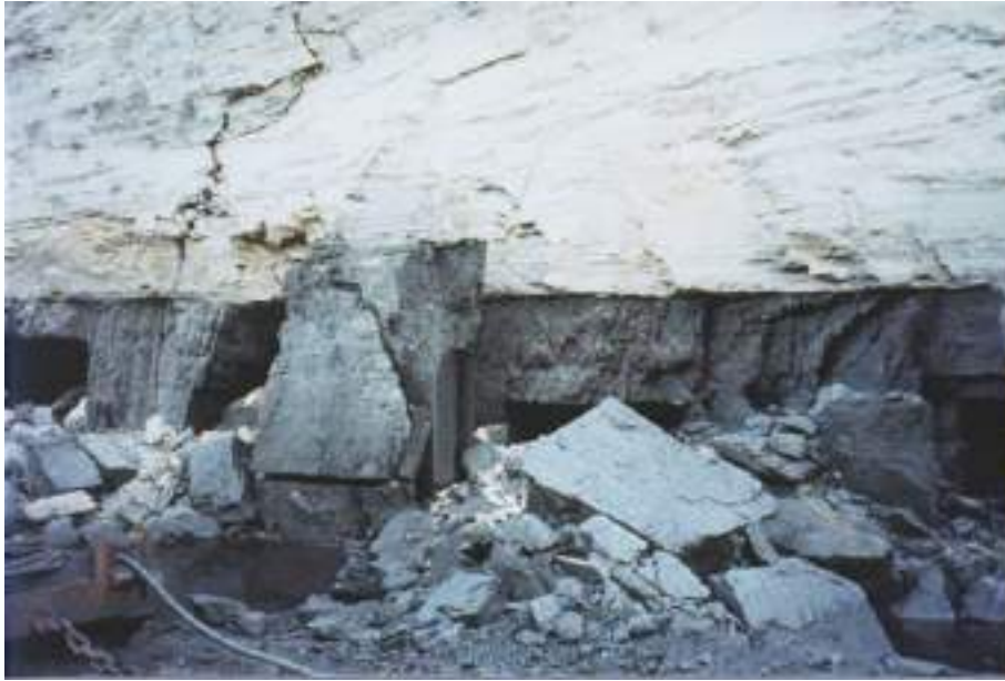
Panel failure – Mine A
