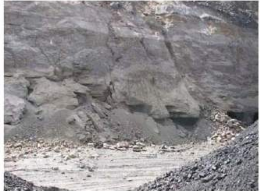
Highwall after failure
