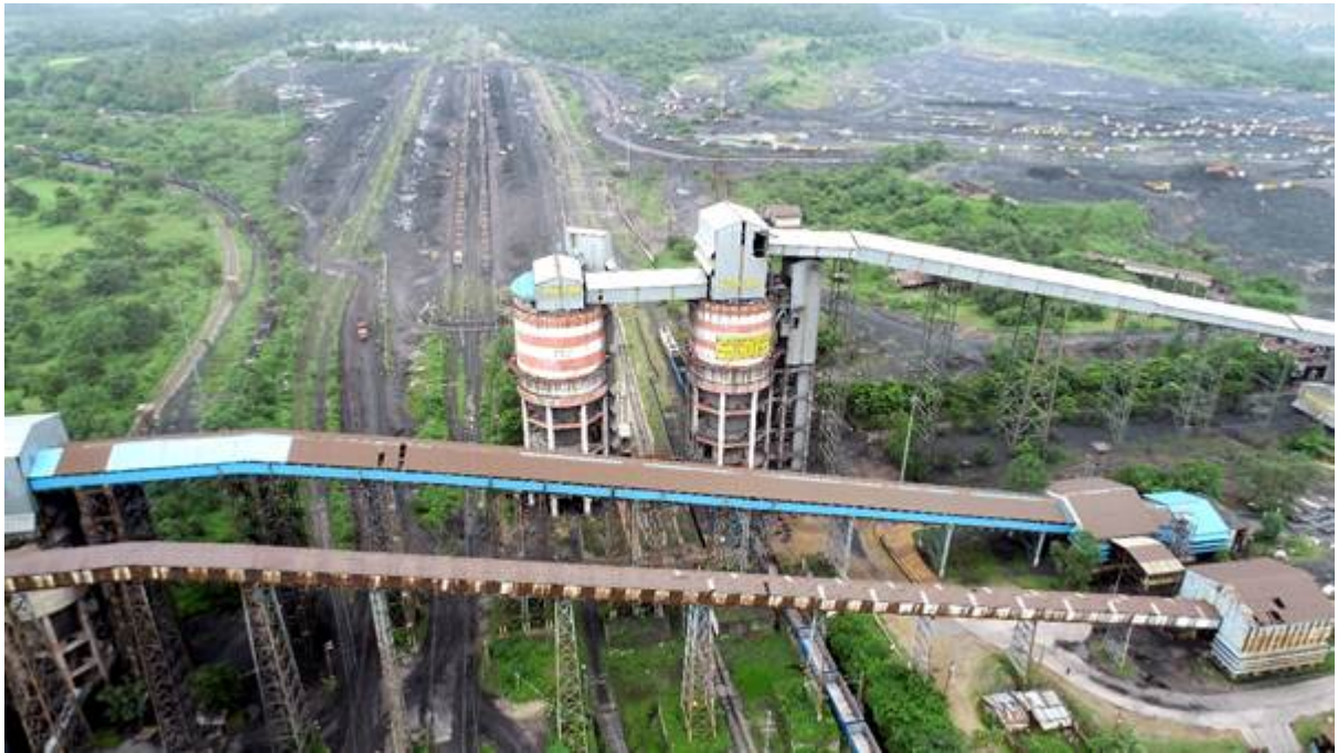
Aerial view of Rapid Loading System (RLS) and Silo under FMC (First Mile Connectivity) at Gevra.
